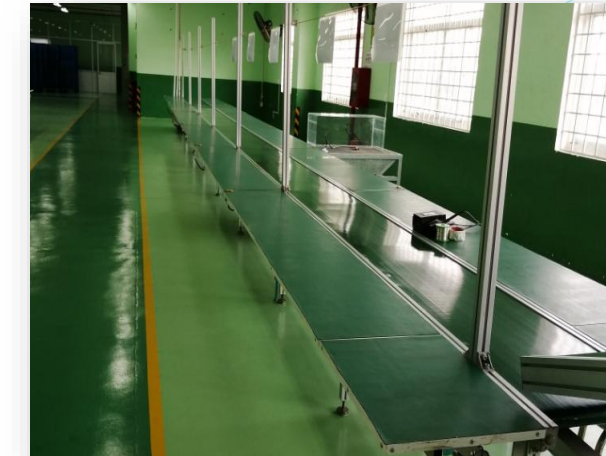
Repair welding 1 line
